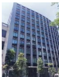
◀ Cross Place Hamamatsucho Minato, Tokyo JPY20.7B/US$180M in May
