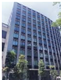
◀ Cross Place Hamamatsucho Minato, Tokyo JPY20.7B/US$180M in May
