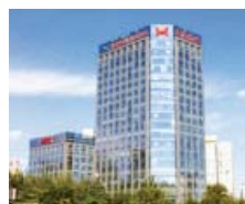
◀ Hainan Airlines Mansion Chaoyang district, Beijing RMB1.3B/US$188.5M in Q3
