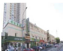
Retail podium of Longzeyuan Western District ▶ Changping district, Beijing in Q3
