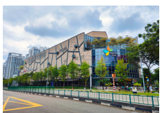
▲ The Seletar Mall 33 Sengkang West Avenue S$550.0M/US$407.9M in March
