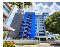
◀ OneTen Paya Lebar 110 Paya Lebar Road S$140.0M/US$103.8M in March
