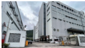
◀ ICI DG Building Tsing Yi, Hong Kong HK$1.08B/US$137.8M in September
