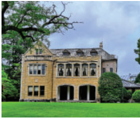
▲ Sanko Kigyō Shirokane Dormitory Site Tokyo JPY50.0B/US$352.0M
