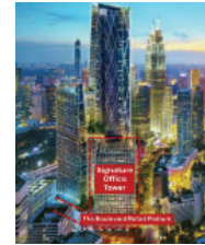
▲ 24 floors (6/F-29/F) of office suites and 4 retail units on G/F & 1/F, Oxley @ KLCC Jalan Ampang, Kuala Lumpur MYR406.0M/US$88.0M in October
