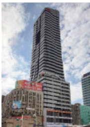
◀ Kee Tai Zhongxiao Building Taipei City TWD12.5B/US$401.7M in October
